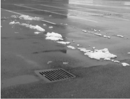
5) Storm drain to the north of stadium receives water not discolored with sediment.
